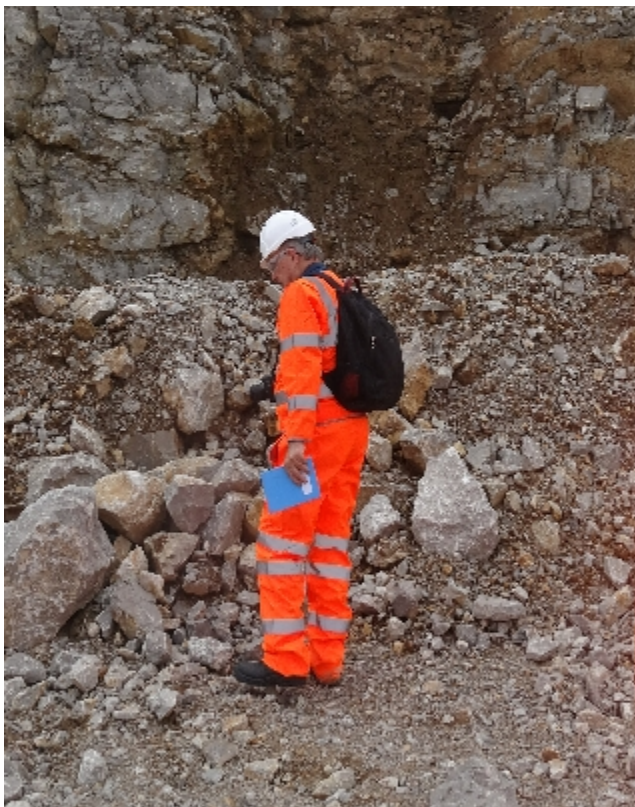
Fig 4. The face bund is lower than the haul road edge bund.
