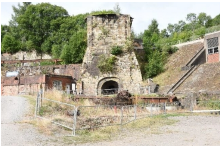
The most recent Brymbo blast furnace
