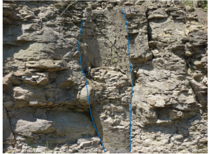
'Tree' in situ , diameter 0.7m approx.
