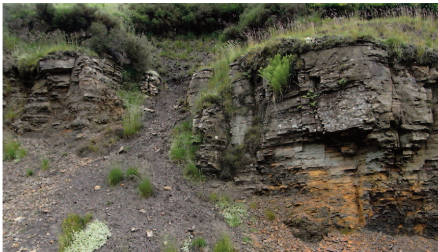
Fig. 4 Cliff section showing the fault.
