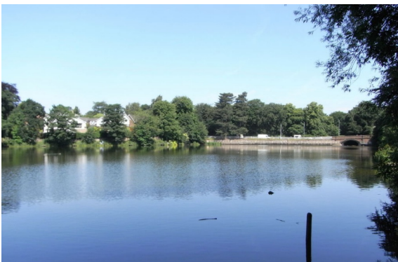
General View of Lymm Dam
