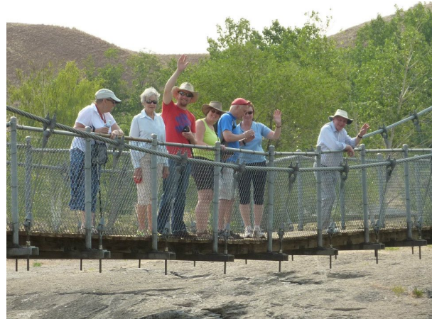
Suspension bridge Thermopolis WY 104° F in shade!!
