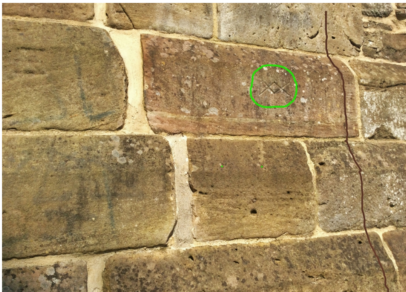
Fig 2 Present day Bridgewater Canal aqueduct and end of the 1822-1824 strengthened and re-faced, buttressed sandstone wall of the original embankment built by Brindley. Photo ©Fred Owen
