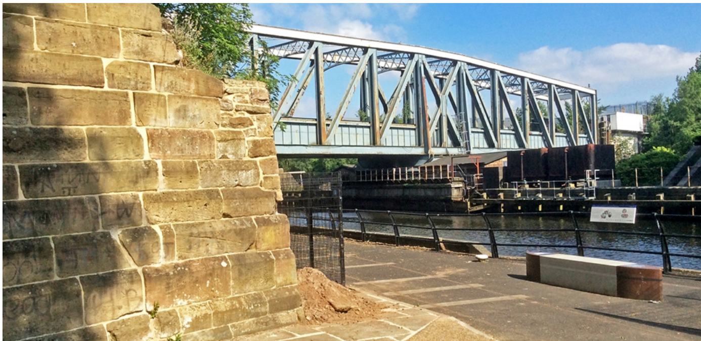
Fig 2 Present day Bridgewater Canal aqueduct and end of the 1822-1824 strengthened and re-faced, buttressed sandstone wall of the original embankment built by Brindley. Photo ©Fred Owen
