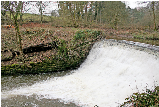
The site of the turbine and fish pass
