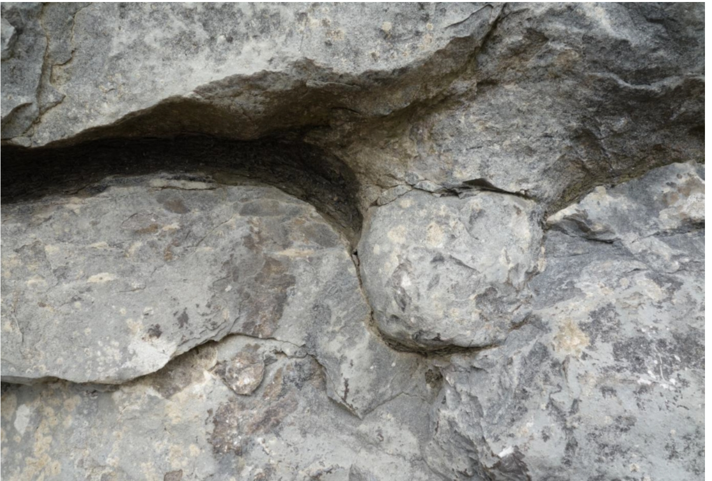
A boss of limestone from the upper unit has penetrated the lower unit; the mudrock parting between the units appears to continue under the boss which is about 200mm diameter
