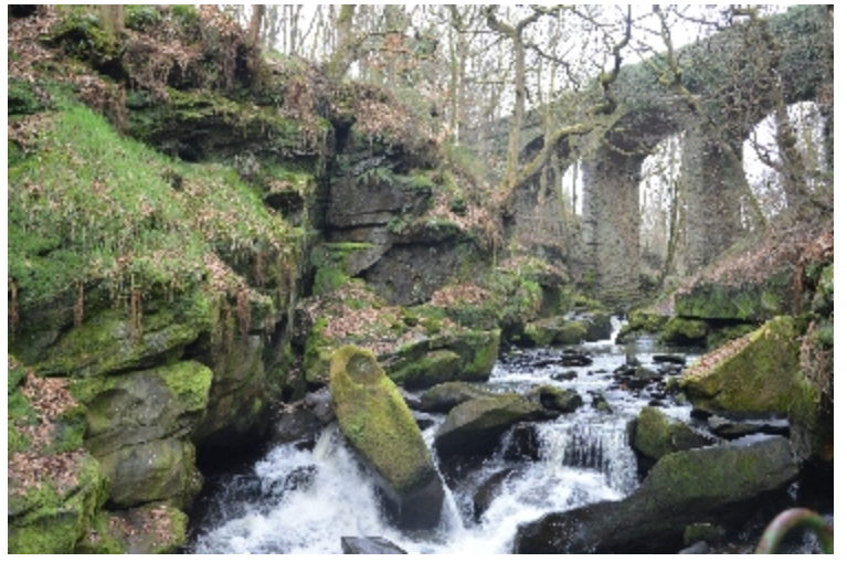
14 Viaduct crossing Healy Dell
