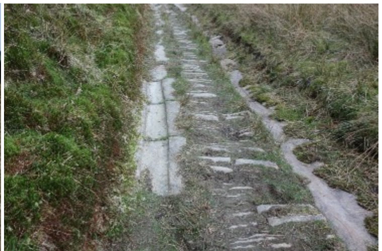
Quarry haul road with wear grooves, perhaps from sledges.
