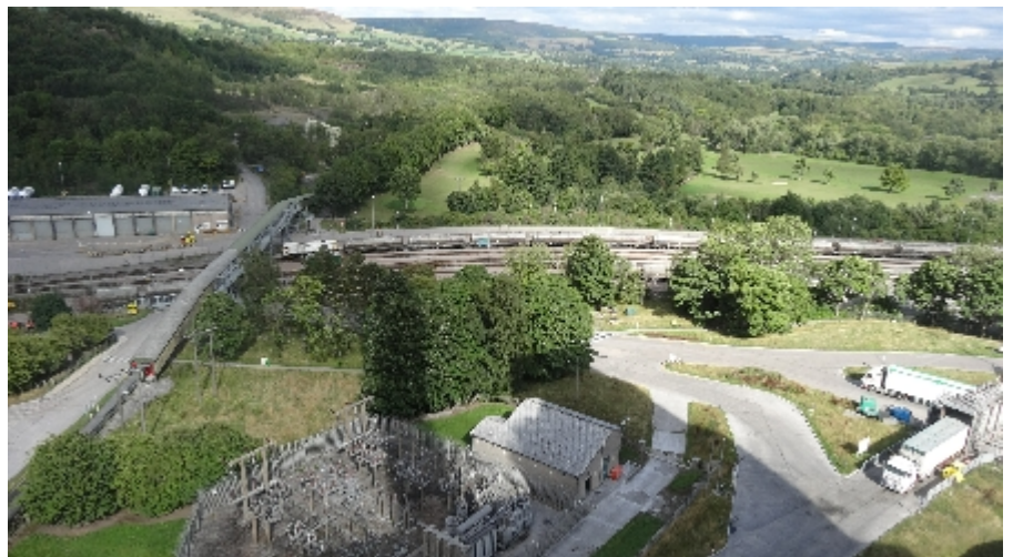
Fig 2. The shale conveyor belt, which is covered as it bridges the railway line is seen to the left of the picture.
