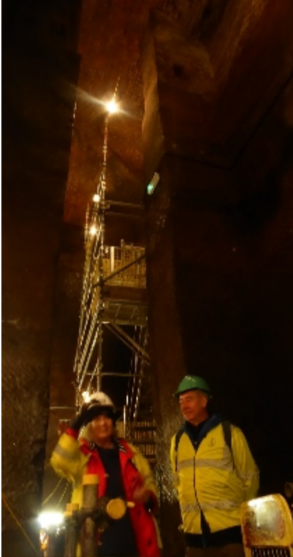
Fig 4 Scaffolding stairways to reach the base of the quarries.
