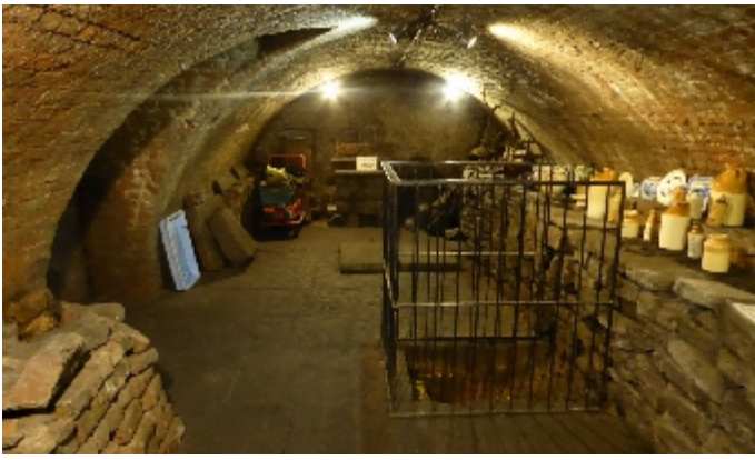
Fig 2 Brick arches had been used to bridge the slot quarries.
