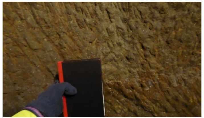
Fig 3 Pick marks on the quarry walls.
