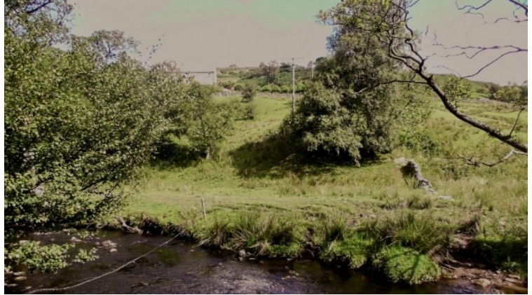
Fig. 1 Signs of landslip on the banks of the river Dane.
