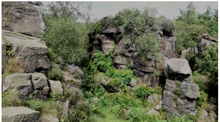
Fig. 6 Rock falls at Castle Rock.
