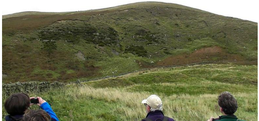
Fig. 7 The Broadlee Bank Tor slip. Note the extent of the area covered and the exposed earth indicating recent slips.
