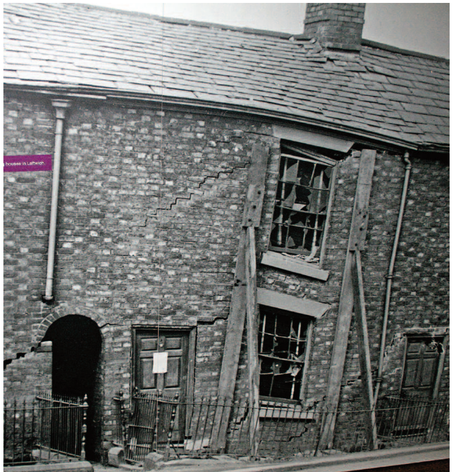
Fig. 4 One result of salt subsidence
