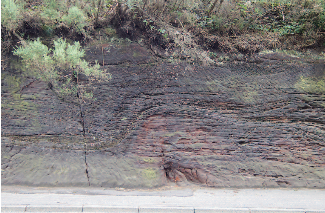
Fig. 1a Bedding in the north side of the A540 road cutting, about 130 metres towards Caldy from the entrance to Thursaston Common Nature Reserve car park.
