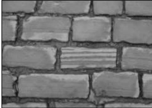
**Figure 18:** Weathered sandstone setts in Lancaster city centre, showing splitting along micaceous partings.
