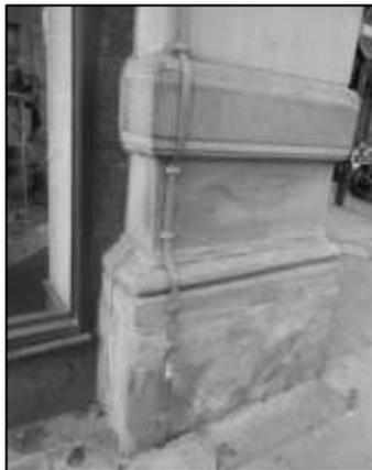
**Figure 19:** Sandstone in Manchester city centre. Spalling probably caused by salt damage.
