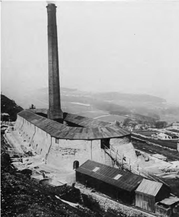
Fig 18: Hoffmann kiln at Harpur Hill, Buxton, courtesy of 'Picture the Past' This kiln has now been demolished
