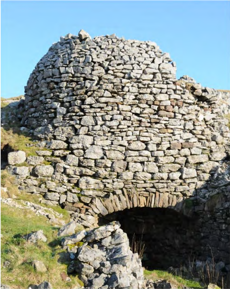
Fig 3: Field kiln near Horton-in-Ribblesdale
