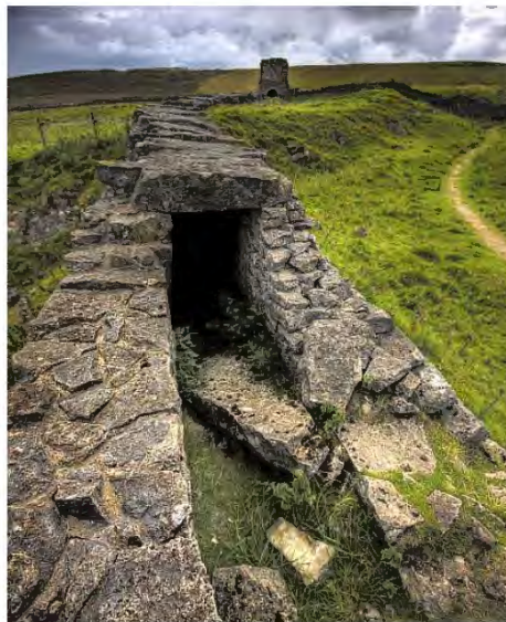
Fig 12: The remains of the flue and chimney stack at Toft Gate. Except when limestone was being loaded to the kiln an iron plate was used to seal the top of the kiln
