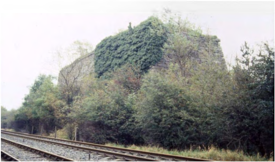
Fig 8: Bank of four industrial scale limekilns near Bellman Quarry. Clitheroe
