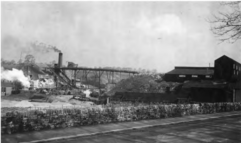
Fig 9: Photograph of the Bellman limekilns in operation. The long bridge-like structure supported an endless chain conveyor which carried limestone and fuel to the top of the bank of kilns (which is to the left of the chimney)
