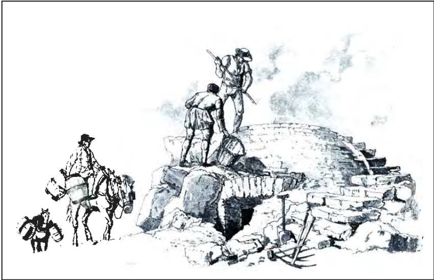
Fig 1: Field kiln with fuel being brought by packhorse (etching from Microcosm , by W H Pyne 1806)
