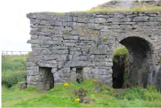
Fig 13: The kiln with coal feeding ports at ground level The quicklime withdrawal arch is lower down at the back
