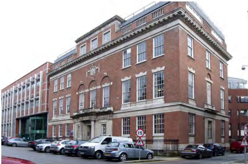
In 2014 the roof space on the 3rd floor has been filled in. The terraced houses to the left are gone, the space now occupied by the National Oceanography Centre. To the rear is the end of the Herdman Annexe, built in the 1980s
