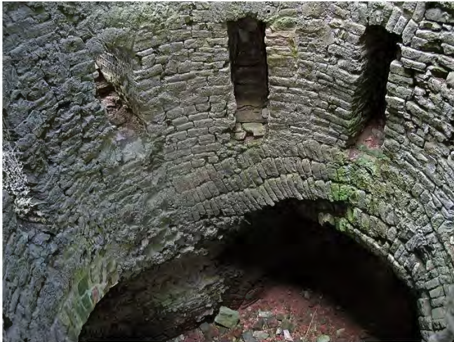
Fig 14: Inside Toft Gate kiln
