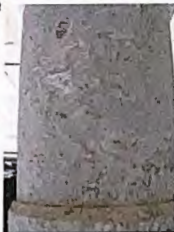
4. On the fountain side of the 5th bollard on the left of the steps (2) Colonial corals originated from a single corallite
