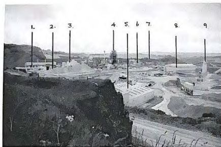
Figure 3. Viewpoint A. Tunstead Quarry. Key: 1. Shaft Kilns. 2. Kiln Feed. 3. Hydrated lime and milk of lime. 4. Maerz Kiln (under construction). 5. Cement Bagging Plant. 6. Aggregate Plant. 7. Old Moor Quarry. 8. Imported materials for Cement Plant: sand, clay, mill scale, gypsum, coal, petcake. 9. Limestone silo for Cement Plant. 10. Woo Dale Limestone. 11. Cement Plant. 12. Chee Tor Rock. I am grateful to Steve Hill, Estate Manager, for information about the plant.
