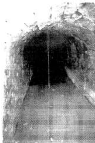
Figure 3. View inside Thornsett Hey tunnel.
